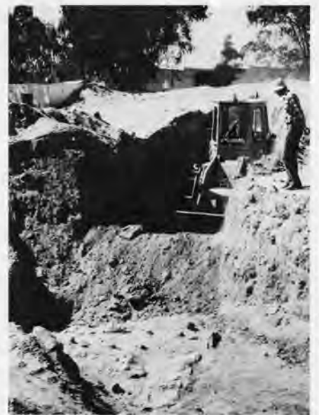
A bulldozer was used to remove over three meters of sand on top of the city wall (visible in the foreground). The location of the Hijaz gate is approximately behind the bulldozer. Photo by D. Whitcomb.
